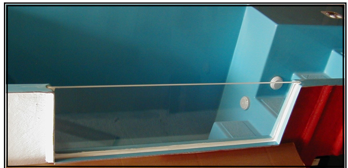
Triple Seal Window Installed
