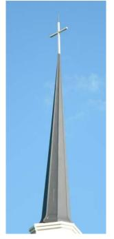
Non—PCT cross shown that rotated 30° and twisted 15° less than 6 months after installation
